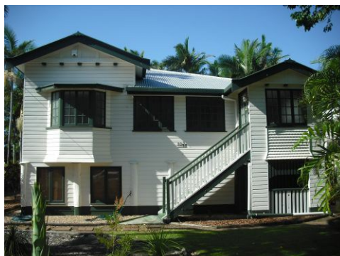
Figure SC6.2.3.10 Illustrates an example of a front façade with projecting gable features
