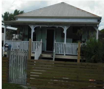
Figure SC6.2.3.8 Illustrates an example of an open front verandah Workers Cottage style
